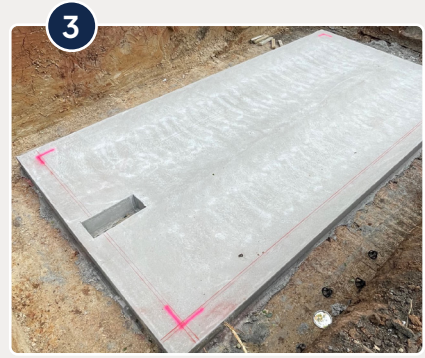
Placement markings on slab, ensure slab is perfectly level
