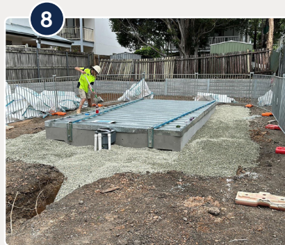
Plungie in place with back fill
