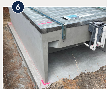
Plungie on perfectly levelled slab
